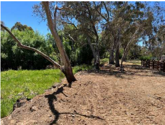
Figure 43. Earthworks in the Barkers Creek riparian corridor
